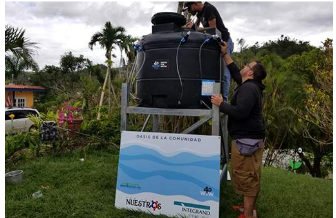
Operational field team installing a water community cistern at Calle Dr. Umpierre ("Los Duros").
